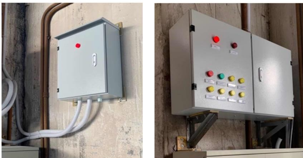
Figure 5. Field installation of signal acquisition and signal transmission equipment.
